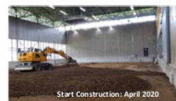
Start Construction: April 2020
