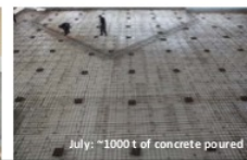
July: ~1000 t of concrete poured
